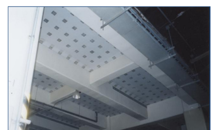
Fig.6 Reinforcement of RC slab with Carbon Fiber Sheet
