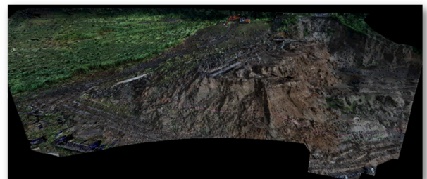
Breached dam body was LiDAR surveyed for its entire 3D image
